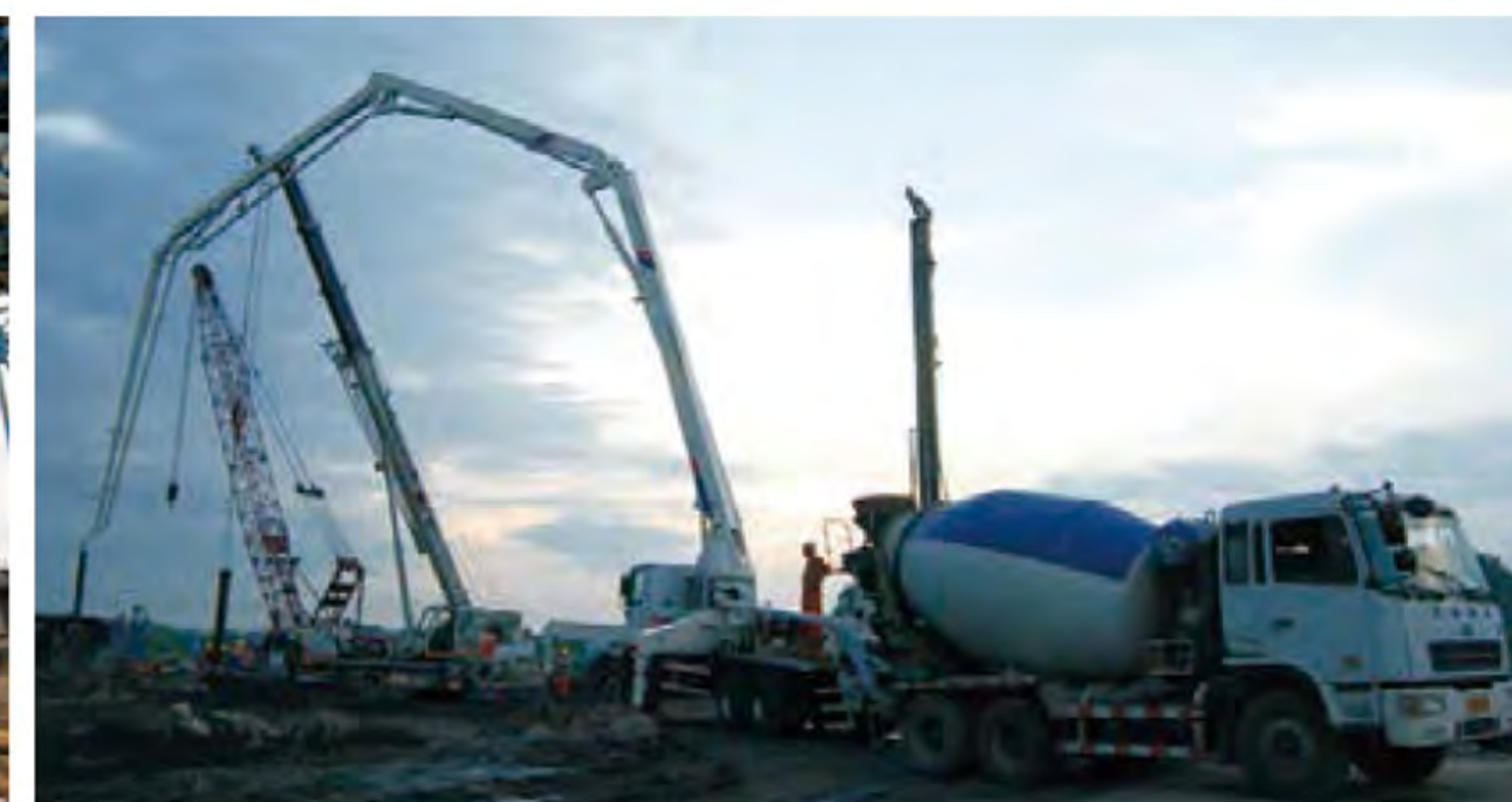
合福高铁施工现场 Hefei-Fuzhou CRH Construction Site
