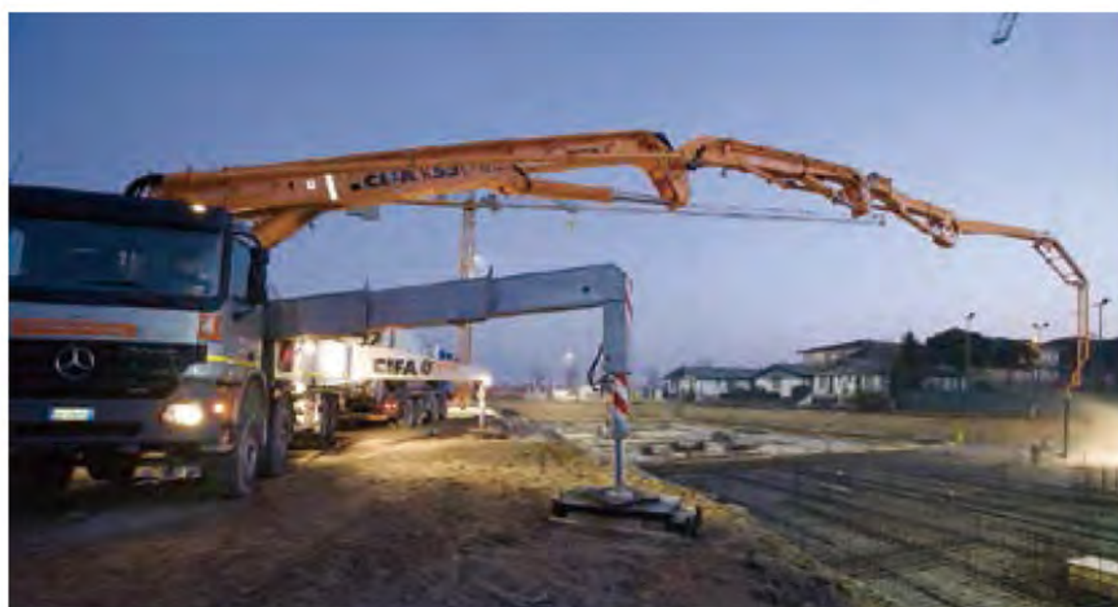
CIFA 泵车意大利米兰施工现场 CIFA Pump Truck at a Construction Site in Milan,Itaiy
