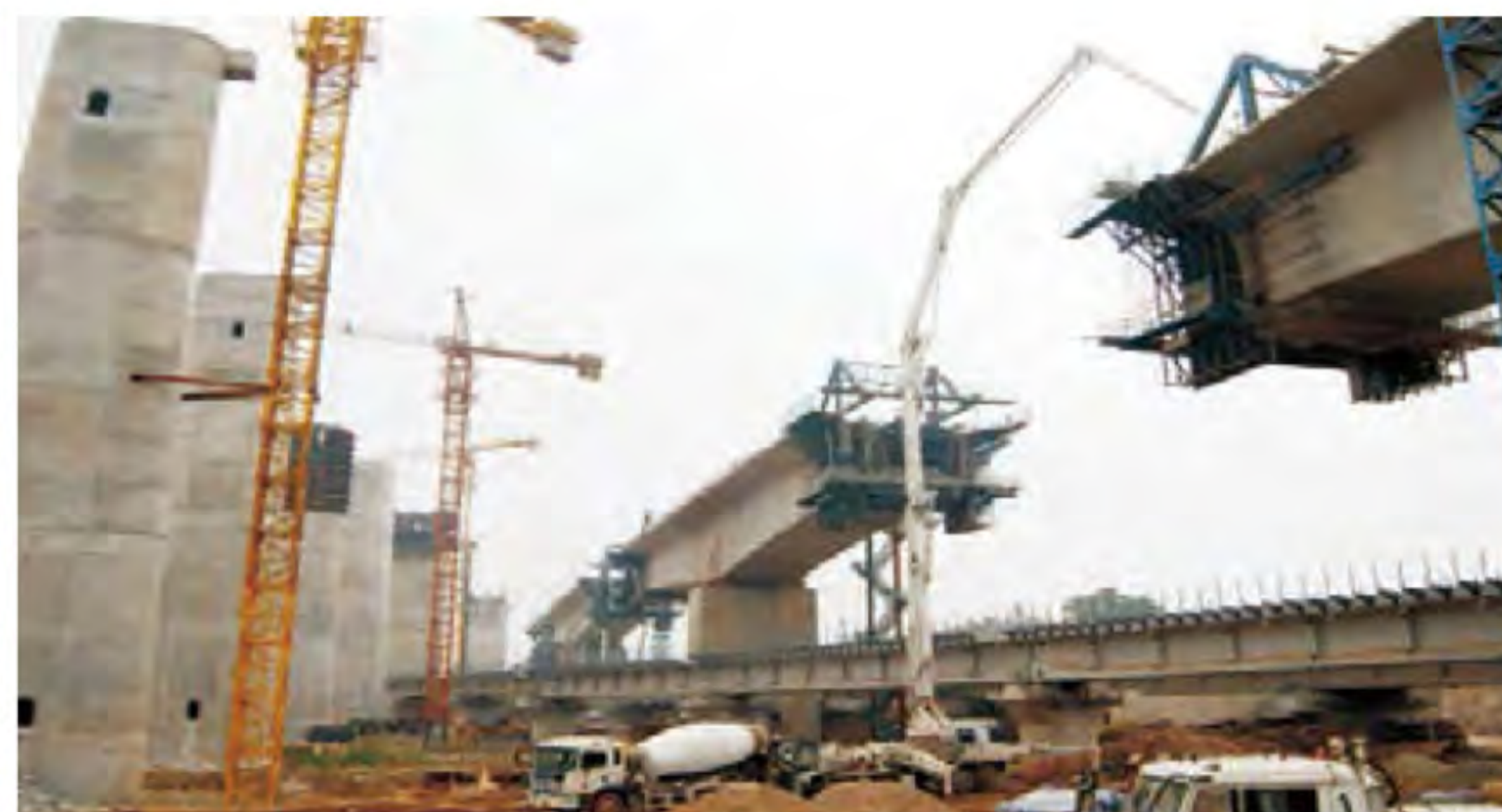
沪宁城际高铁施工现场 Shanghai-Jiangsu CRH Construction Site
